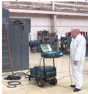
Pf Testing of Capacitor Bushings
